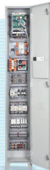
STEP Elevator Serial Integrated Controller
